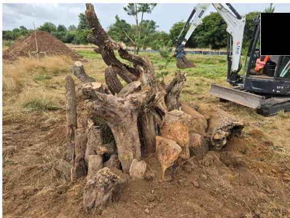
Image 22: Vertical log piles
